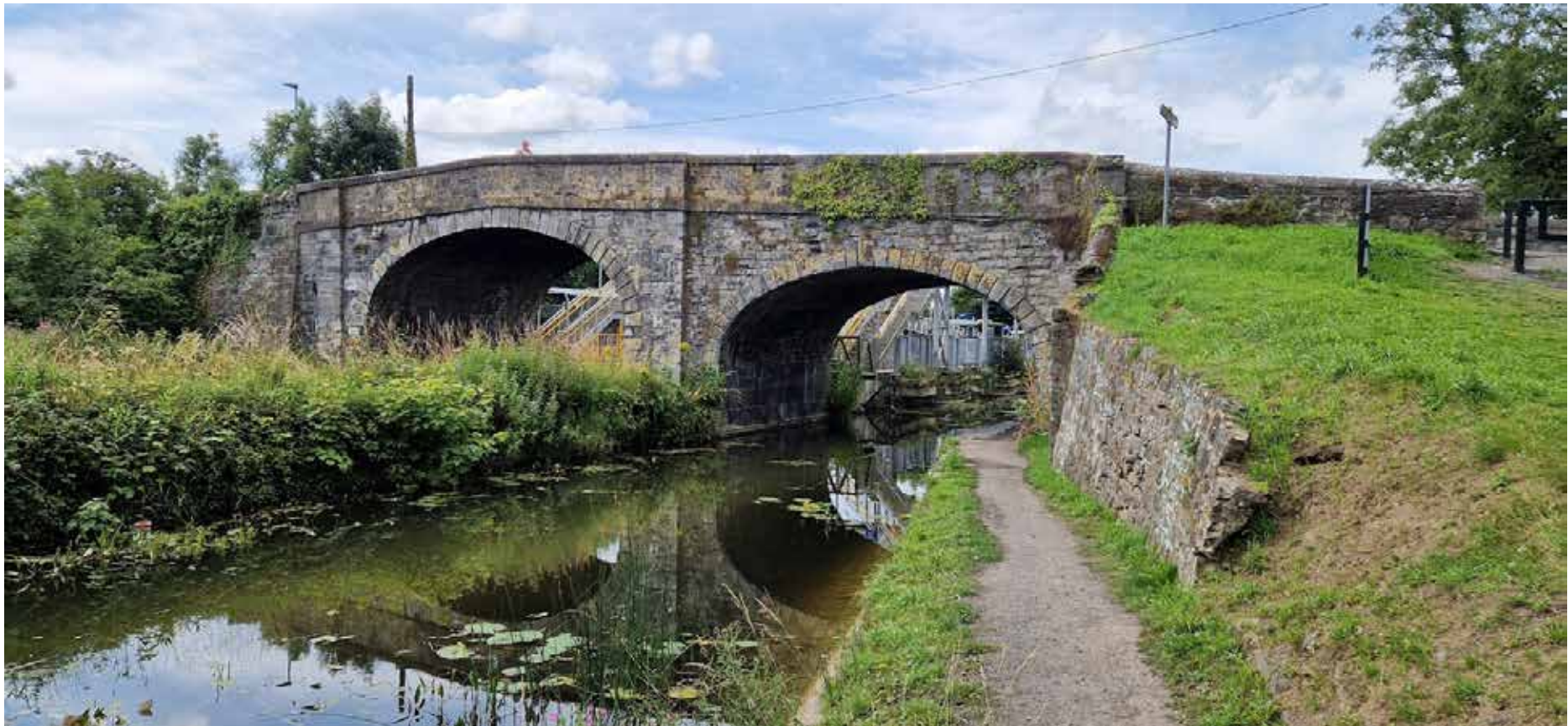
View of the Leixlip Bridge with the Leixlip ( Confey) Dart Station beyond
